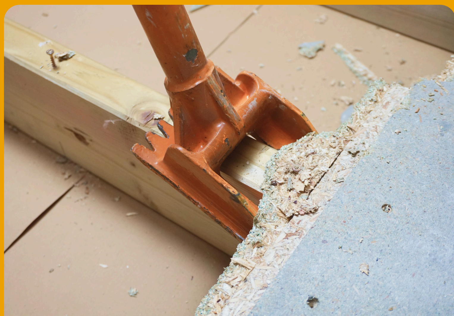
Straddle the Joist
