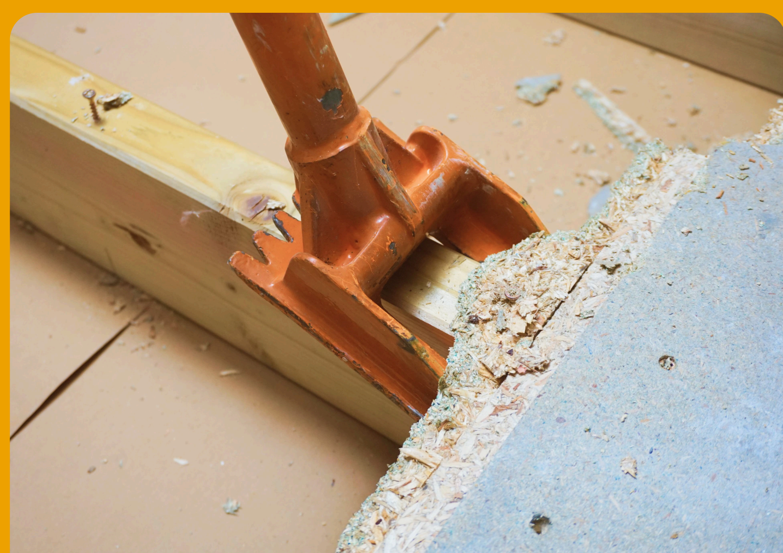
Straddle the Joist
