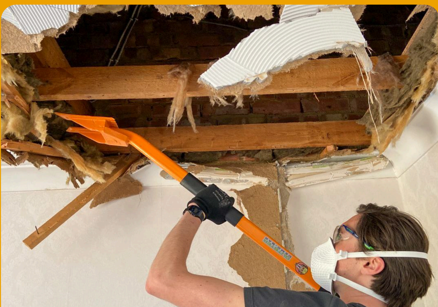
Straddle the Joist
